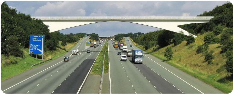
M1 motorway in Yorkshire
